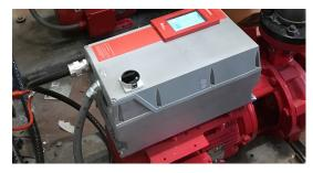
Armstrong maps each individual pump's hydraulic, motor and inverter variations at the factory, to achieve exceptional accuracy throughout the flow range. With this calibration, Armstrong Design Envelope pumps also serve as flow meters, providing reliable system flow data (+/- 5%). The testing ensures optimal performance efficiency at start-up, and Armstrong's Pump Manager helps maintain and extend efficiency throughout the pump's operating life.
